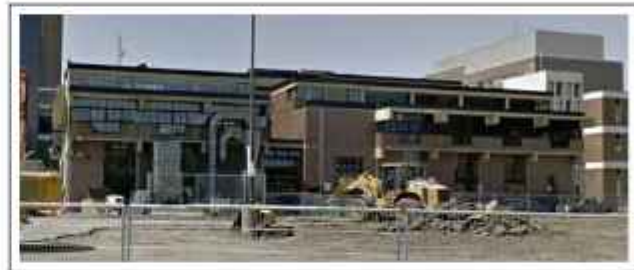
Figure 4. Architecture Building east façade, 2018—Starting of construction phase.
